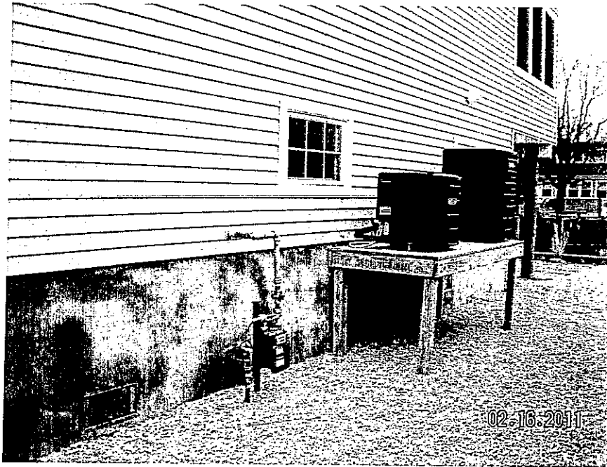
116 Bonita Road, A/C UNITS
